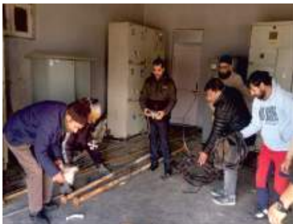
Cleaning near generator room
